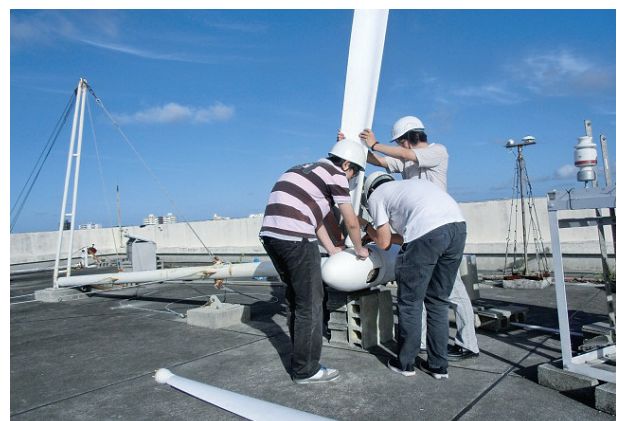
3kW horizontal wind turbine generator with three variable pitch blades
